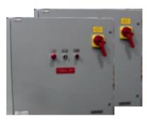
The CU2 units consist of standardized contactor units to sequence CEP system operation according to presence/absence of grid power.
